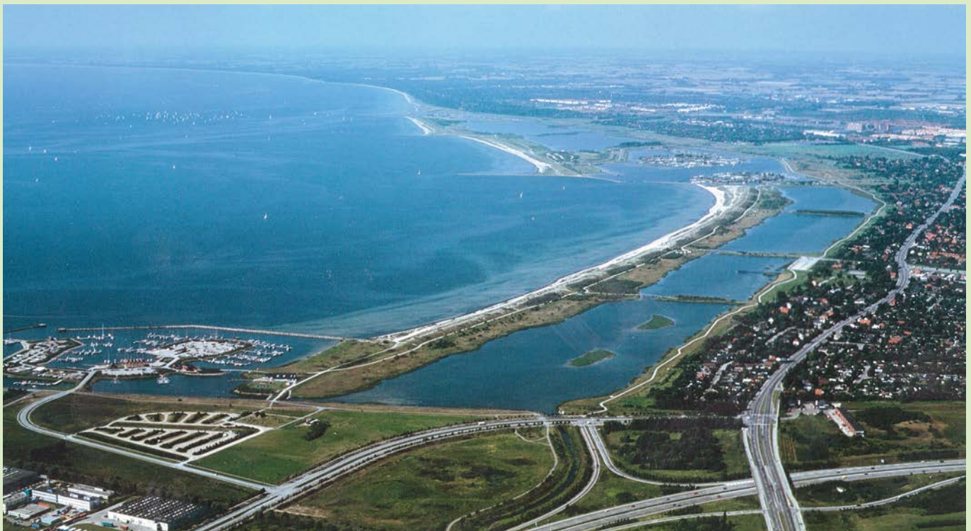
Køge bay Beach Park, Denmark: A scheme which combines flood protection, recreational beaches and marinas. A dike is hidden in the man-made dunes and runs around the marinas protecting the hinterland (From CEDA Information Paper (2012): Climate change adaptation as it affects the dredging community. Available on www.dredging.org )
