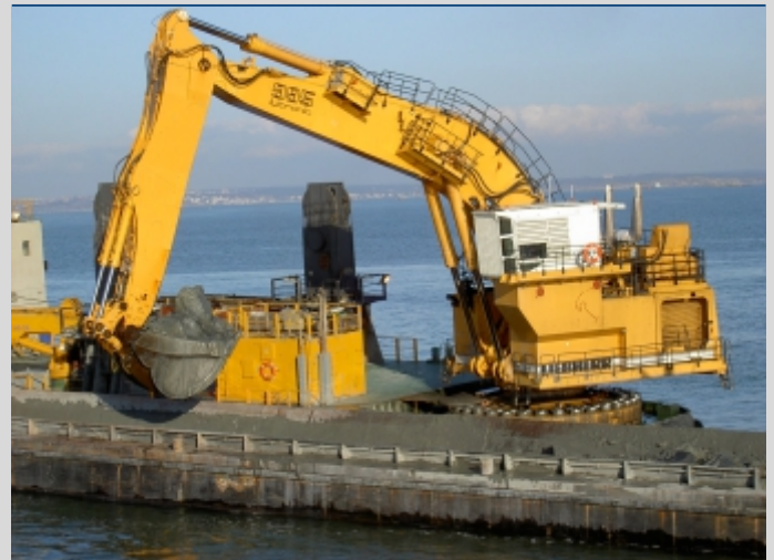
BHD Loading barge
