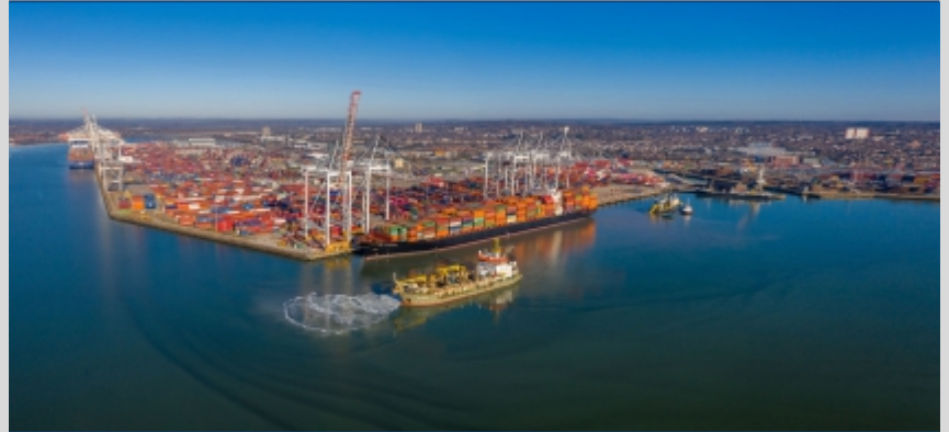
Maintenance Dredging - Southampton Port (source: Boskalis)
