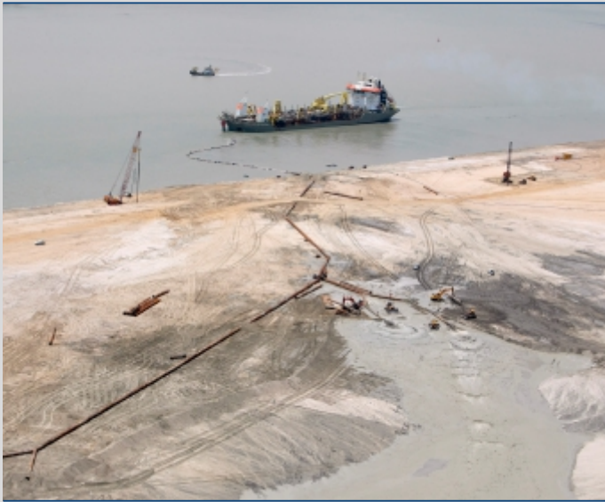
Reclamation- Port Tanjung Pelapas, Malaysia (source: Boskalis)
