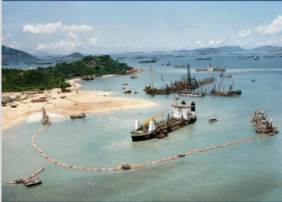
Capital Dredging - Hong Kong
