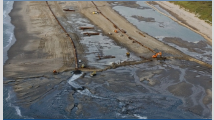
Beach Nourishment- Hondsbossche Zeewering (source: Dredging for Sustainable Infrastructure )
