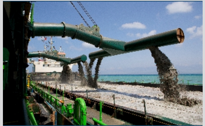
CSD loading barge (source: DEME)
