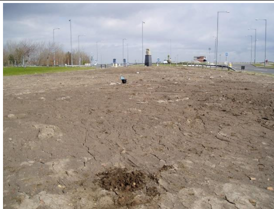
Figure 2. Baseline sampling after dewatering, April 2008.
