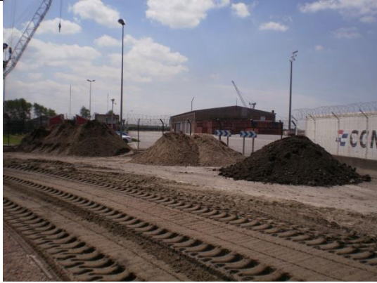
Figure 1. Pre-treated sediments used in sub base road layers (left) and application of hydraulic binders (right)
