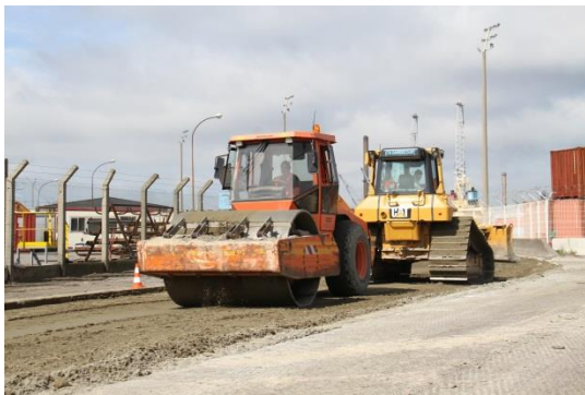
Figure 2. Leveling and compaction of the sub base road layer
