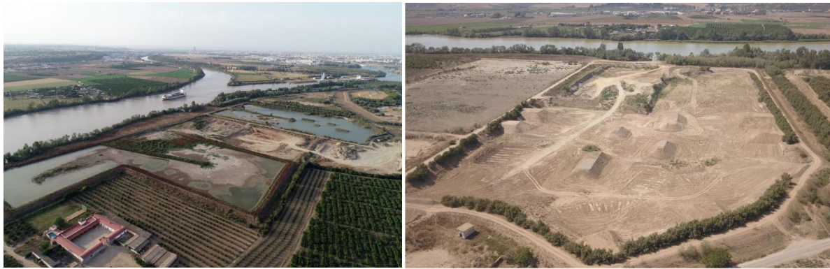
Figures 1 and 2. Aerial view of the Port of Seville's land-based disposal facility adapted by creating islets and dikes to encourage bird breeding. Butano's disposal area under construction.
