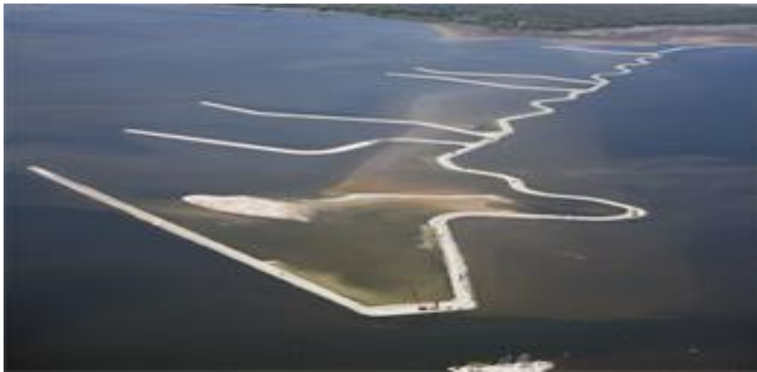
Figure 2. Constructed wave barrier in 2011
