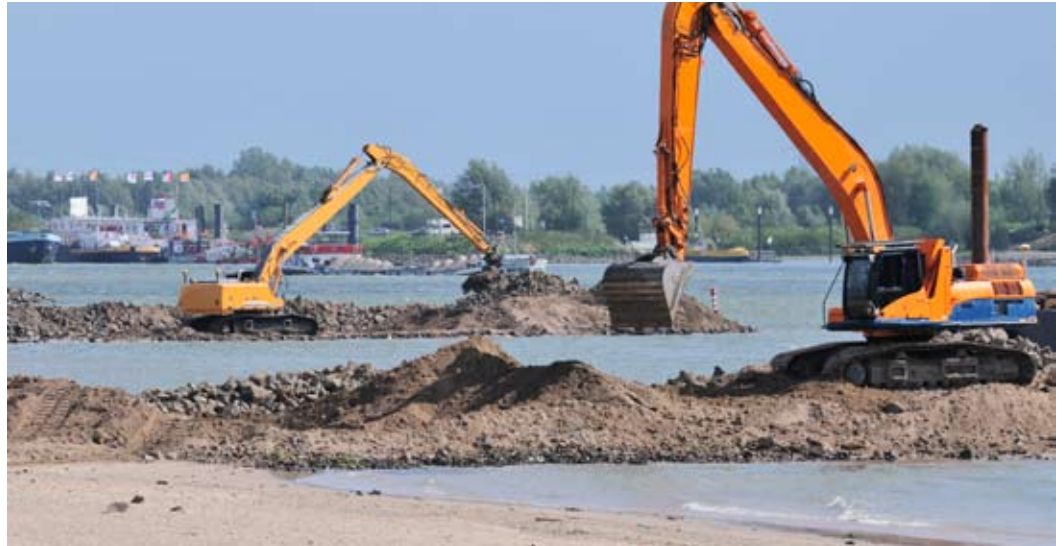
Work in progress lowering groynes
