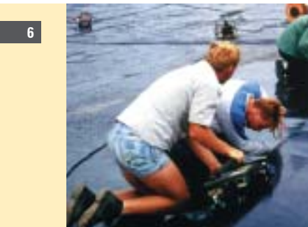
Welded sheets of PEHD plastic are laid as a basic seal to prevent dispersion of contaminants, at the Francop land-based CDF in Hamburg, Germany.
